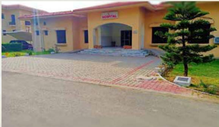
Outer View of College Hospital
